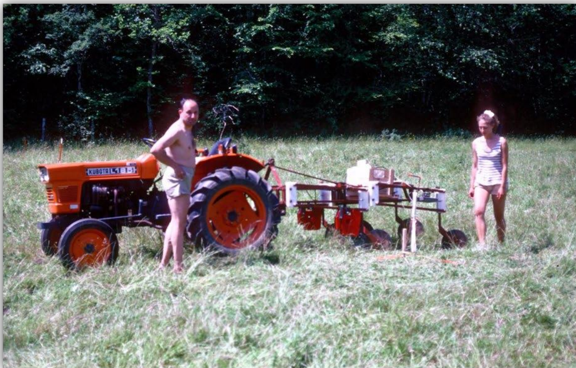
Figure 13. During Michel Dabas' PhD, in 1986, he was developing with Albert Hesse, Alain Tabbagh and Alain Jolivet (pictured in front of the tractor) the first automated system for resistivity mapping (description and picture taken in Minot-Brevon provided by Michel Dabas).
